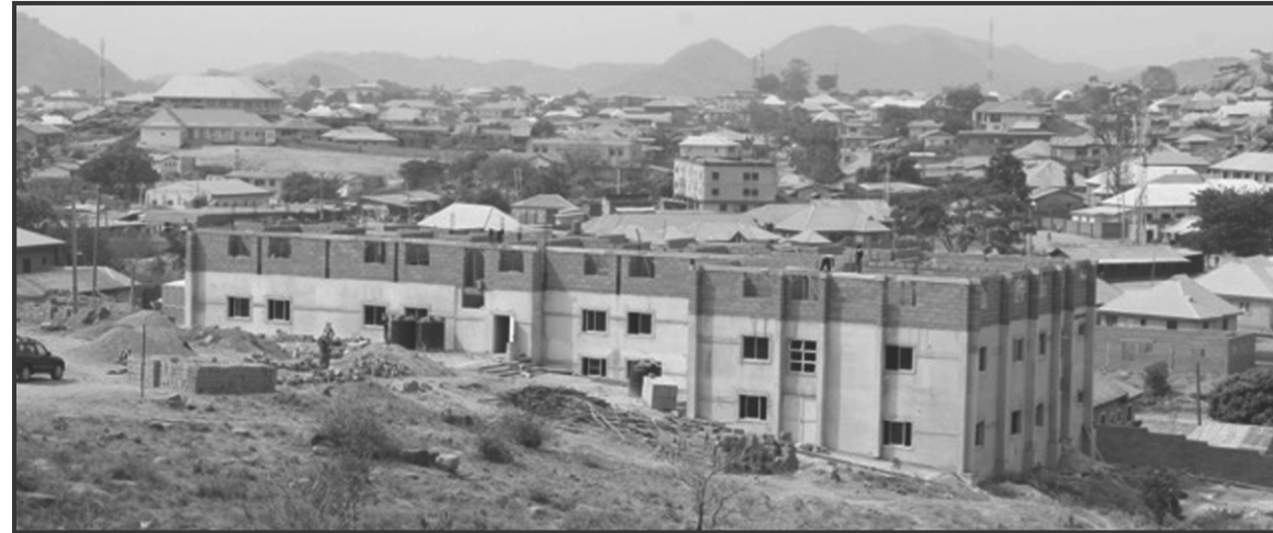
Pouring the lentils for the second floor
