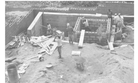
Construction of Septic Tanks
